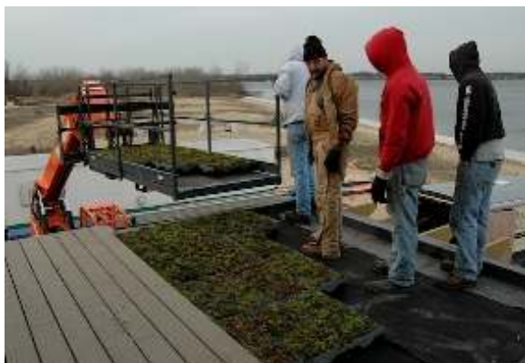
"Green Roof" installation at a lakefront condominium development in Muskegon
